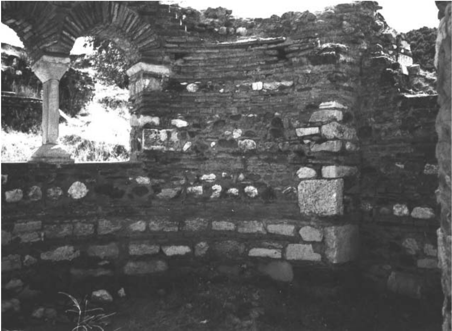
SARDIS. View from inside the church building.
