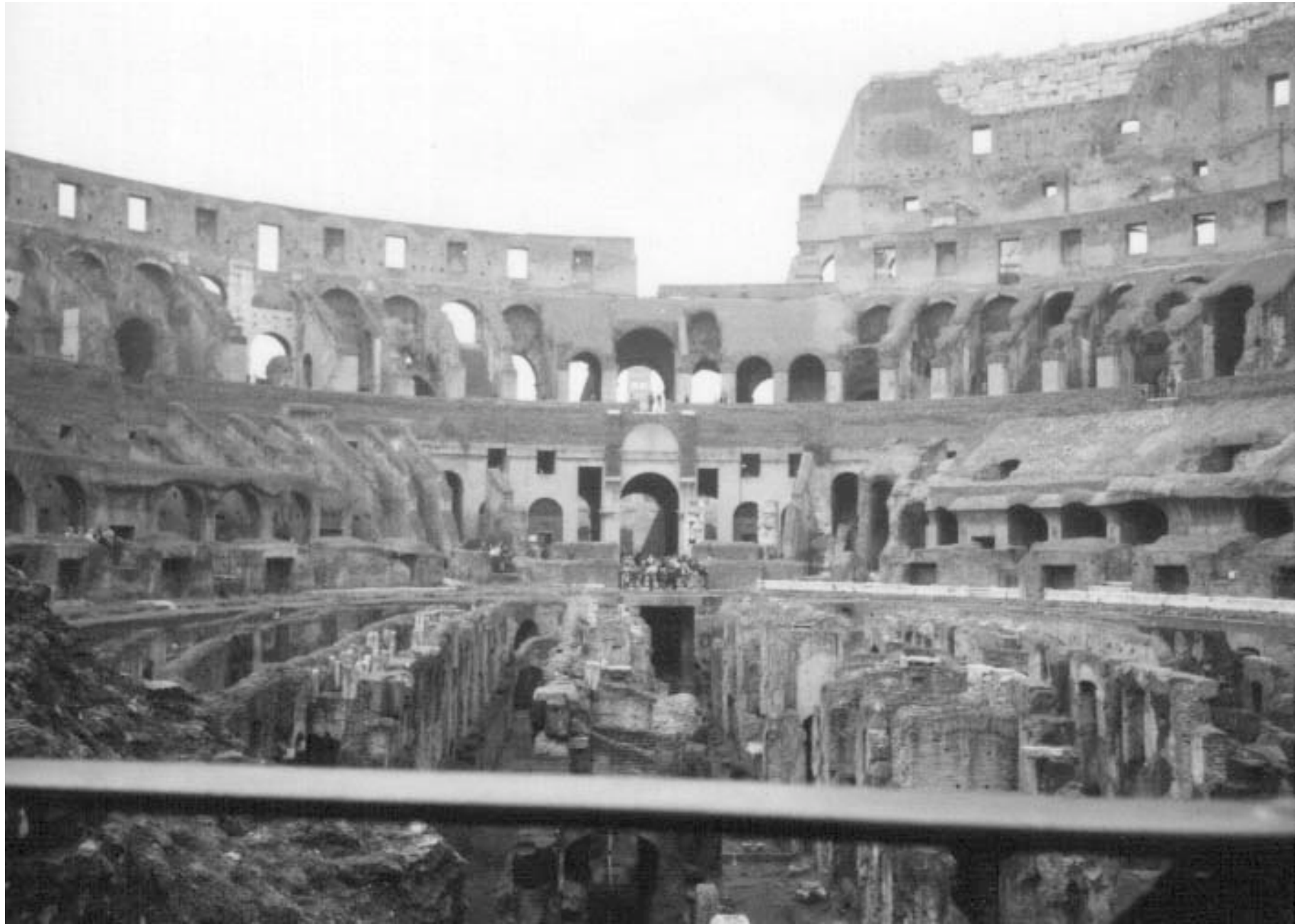
ROME: View inside the Colosseum, revealing the passageways located underneath the floor (which is missing), where wild animals, gladiators, and others were kept prior to their "contests."
